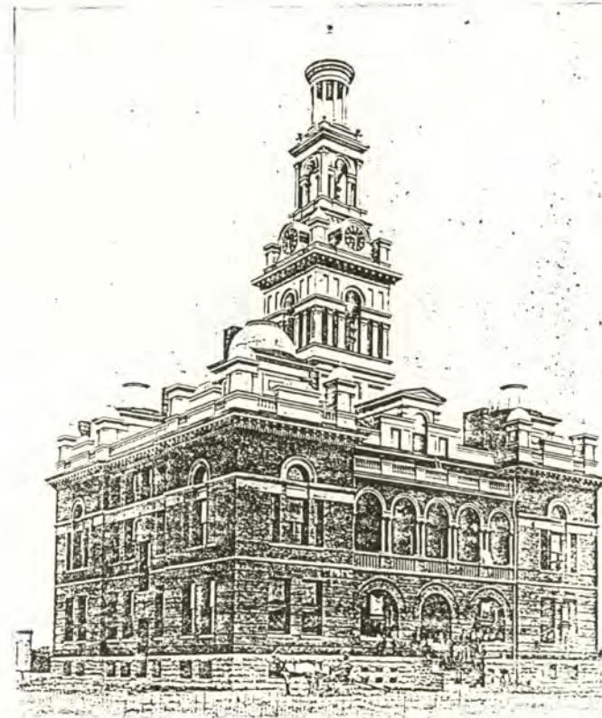
Sevier County Court House, Sevierville, Tennessee, 1896.
